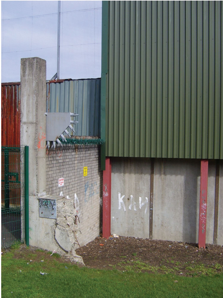
Figure 3. The peace wall at Falls Road / Shankill Road showing the joins where different phases of peace walls meet.
